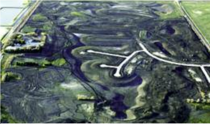
Ariel view shows work on the new Crow Wing golf & residential development at Niverville.
